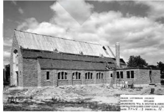
Image 18: July 19, 1959, roof wood plank sheathing in progress. South elevation. Source: Grace Lutheran Archives, Construction Scrapbook.
