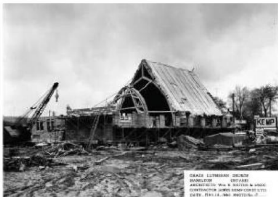
Image 15: May 1959, exterior walls and the structural laminated timber in progress. Source: Grace Lutheran Archives, Construction Scrapbook.
