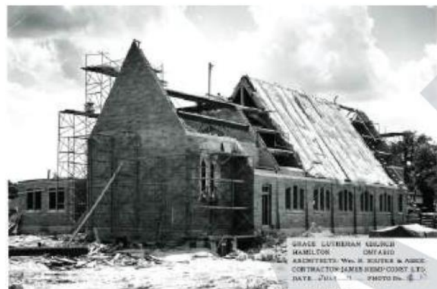
Image 16: July 4, 1959, exterior walls, structural laminated timber and structural concrete block and limestone wall at alter in progress. Source: Grace Lutheran Archives, Construction Scrapbook.
