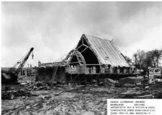
Image 23: May 1959, exterior walls and the structural laminated timber in progress. Source: Grace Lutheran Archives, Construction Scrapbook.
