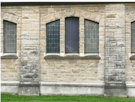
Site Photograph 16: Note trim around windows and smooth limestone windowsill and base around church. Photo Credit: Don Loucks.
