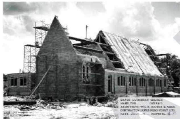
Image 24: July 4, 1959, exterior walls, structural laminated timber and structural concrete block and limestone wall at alter in progress. Source: Grace Lutheran Archives, Construction Scrapbook.
