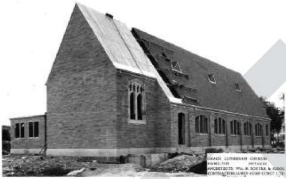
Image 25: July 11, 1959, roof wood plank sheathing in progress. North elevation. Source: Grace Lutheran Archives, Construction Scrapbook.
